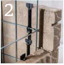
Use connector to attach Lafitt Tandem Veneers to grid
